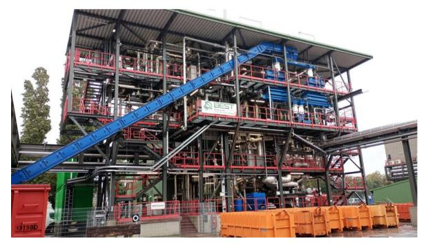
The 1 MW advanced dual fluidised bed gasifier in Simmering produces a nitrogen free syngas suitable for making synthetic fuels.
