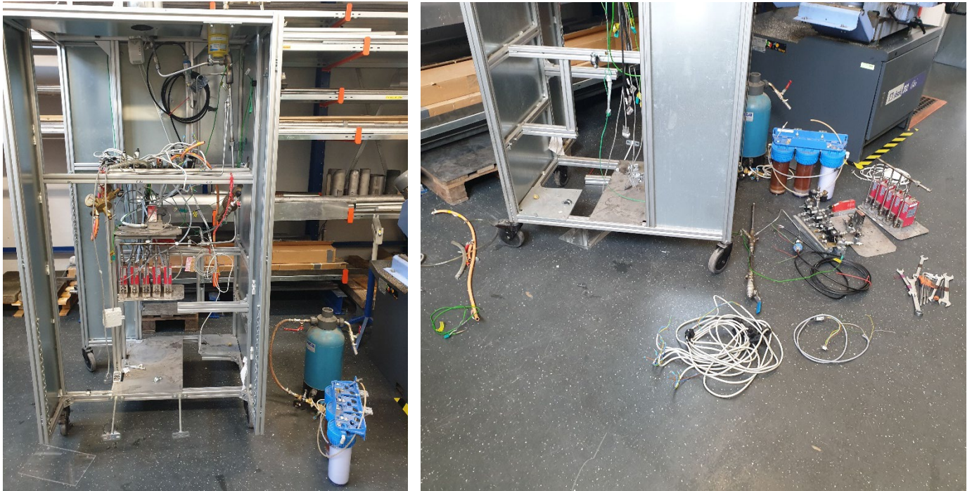
Figure 13: Dismantling of the old gas mixing station
